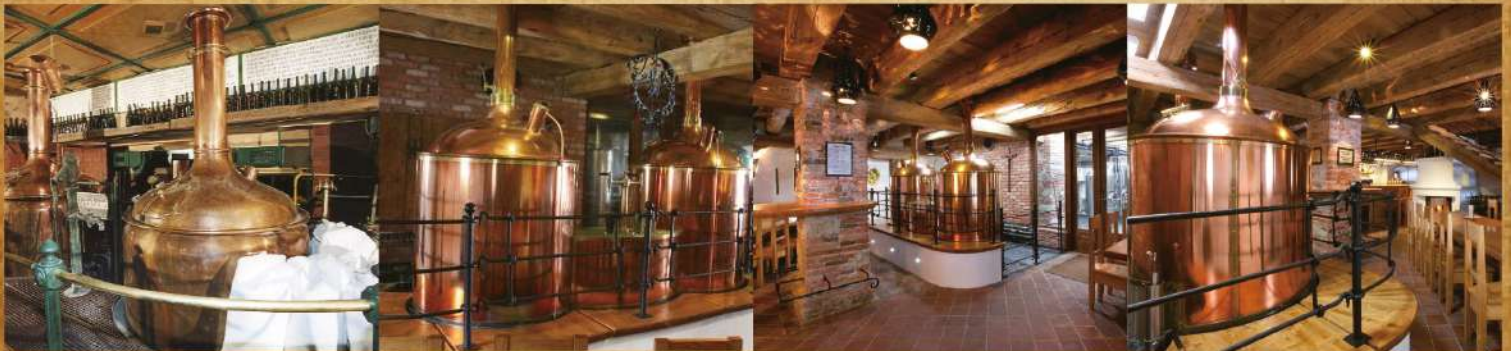
Beer system as a part of interior design in Czech pubs , reference pictures were used
